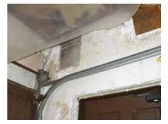
Here's some exposed foam insulation inside an attached garage that should be covered with drywall
