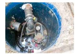
Sump pump at exterior, note high water level alarm float at discharge
