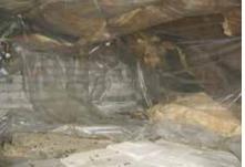
Here's a poorly installed vapor barrier on the ceiling of the crawlspace instead of the floor where it should be located.
