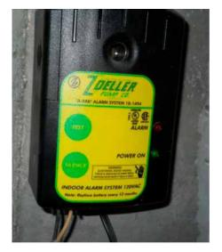
*High water level alarm with battery backup. Connects to a float in the sump.*
