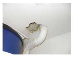
As you go into the garage, be clear as to exactly what parts of the garage connect to living space. Is it one wall, two walls, three walls? Is it all or part of the ceiling? Look for areas where the tightness of the wall may have been breached or where inappropriate materials have been used.
