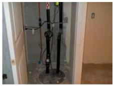
Sewage ejector in basement closet. Note check valve at discharge and shutoff
