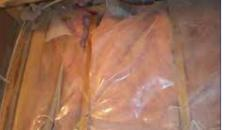
Damaged polyethylene film such as this is an ineffective vapor barrier, and an even more ineffective air barrier
